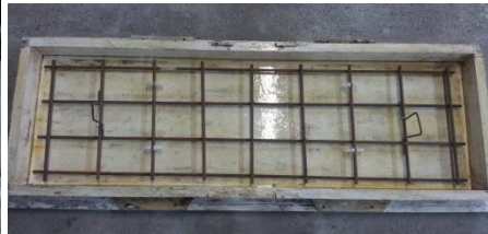
b: Steel cage erected inside mould
