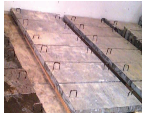
f: Slabs after curing
