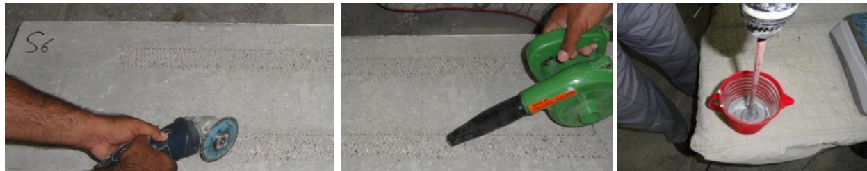
a: Removing the weak layer surface
