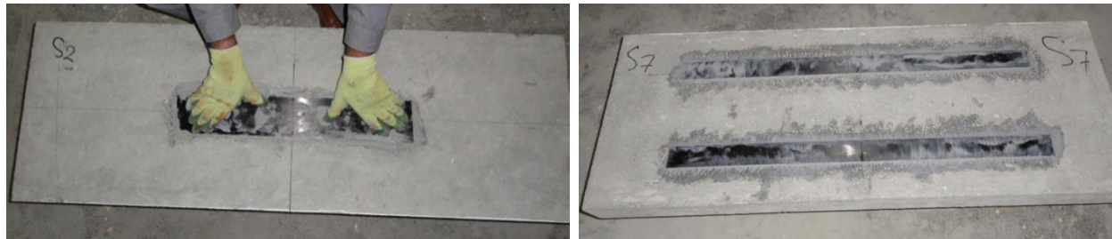
d: Applying of CFRP strip
