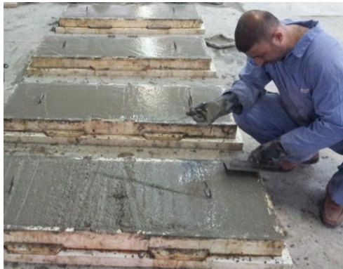
d: Concrete casted in moulds
